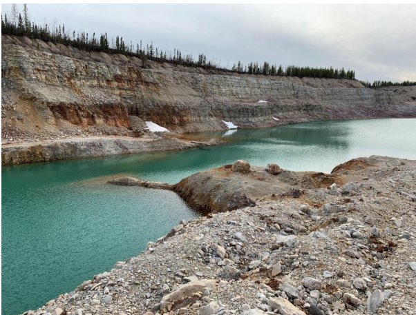
Photo 1: View of existing open pit N42 at the historical Pine Point Mine site.
