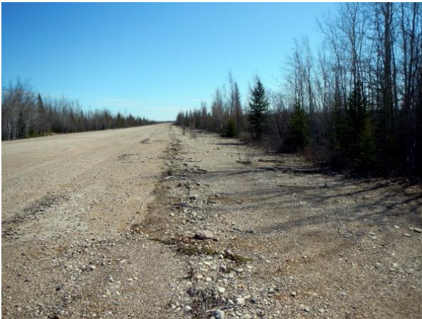
Photo 3: View of existing haul road at the historical Pine Point Mine site.
